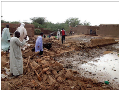
Abalak houses collapsed after the 23rd August storm and floods
