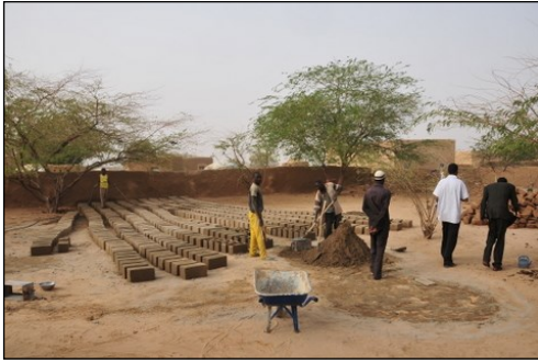
Beginning construction of the Primary School in March 2009
