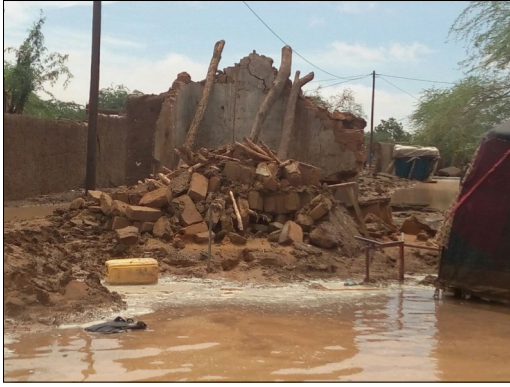
Collapsed house in the area of TANAT school.
