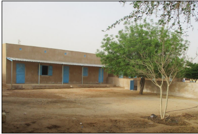
The new Nursery School building ready for the October 2019 commencement. As standard dictates, the building is physically separated by a wall from the rest of the primary school.
