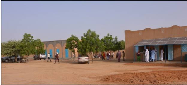
The administrative building with its solar panels made porch roof, the computer room and the library of the secondary school.
